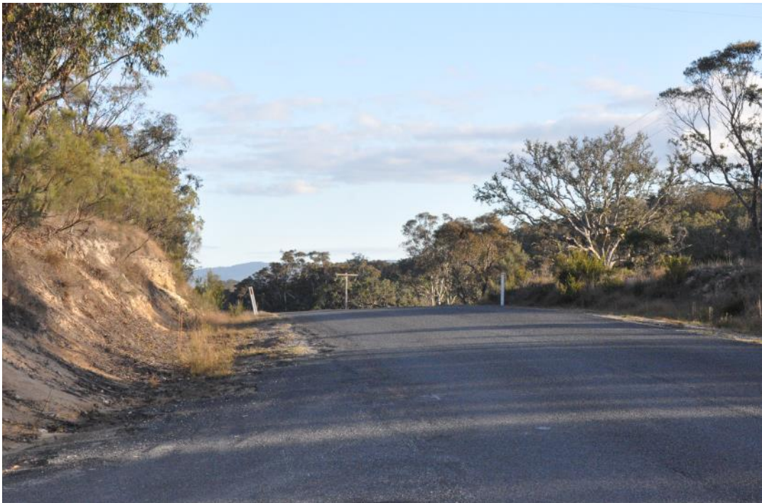
Plate 3 Poor sight distance due to crest looking south at Bryans Gap Road
