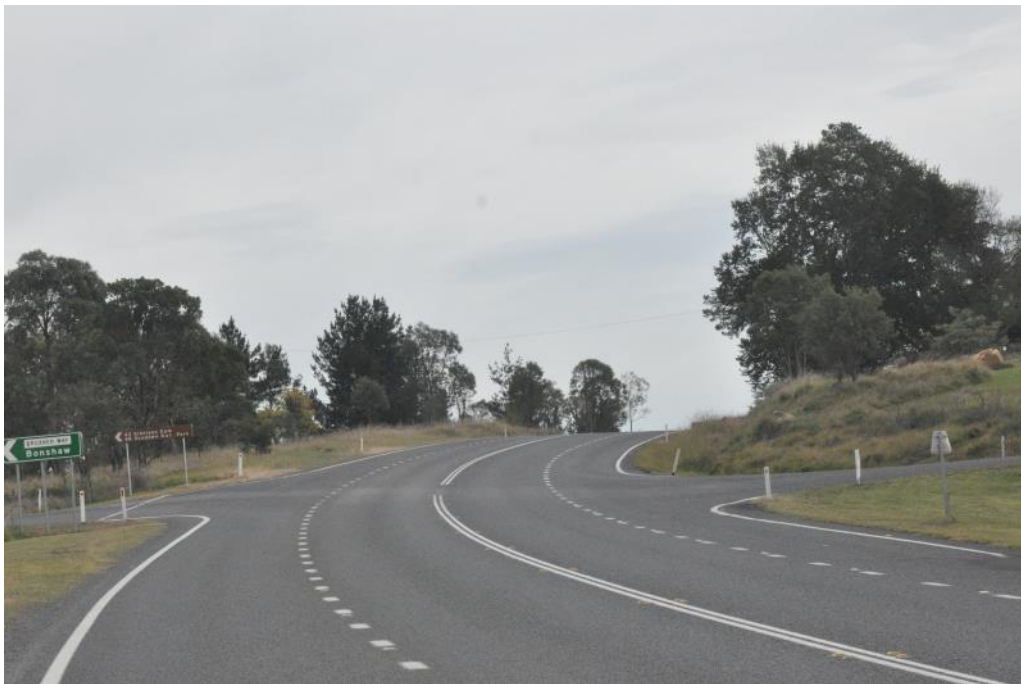
Plate 4 Poor Sight Distance due to crest looking north along the New England Highway
