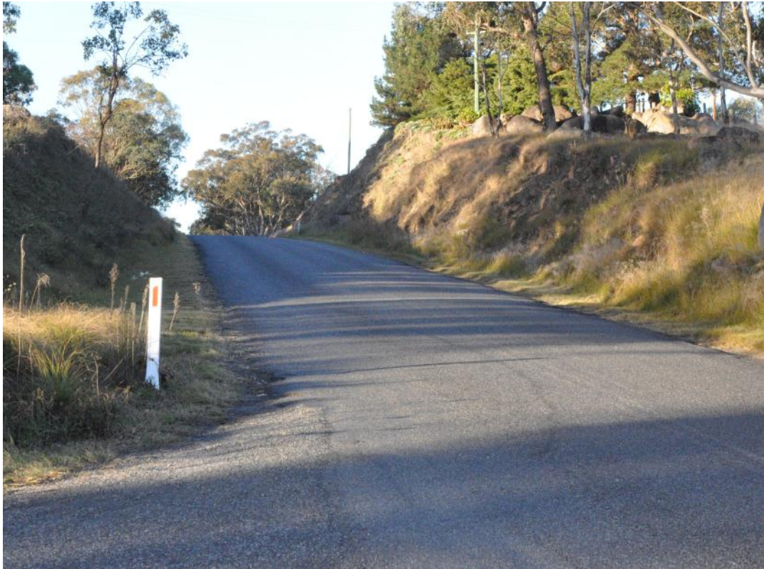
Plate 2 Poor sight distance due to crest looking north at Leechs Gully Road Intersection
